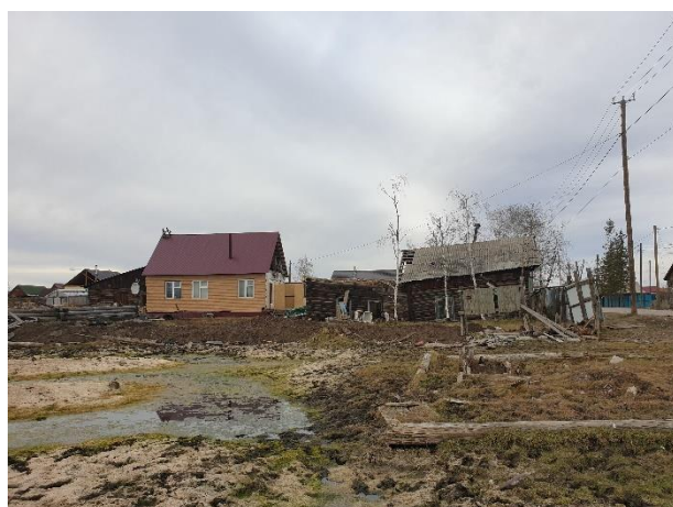
Fig. 15. Abandoned and new houses on the site damaged due to the activation of thermokarst on the site in Amga, September 2021. Photo by A.A. Suleymanov.
