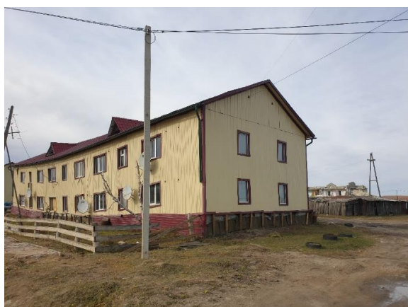
Fig. 18. Apartment building on the Mira Street, affected by thermokarst.
