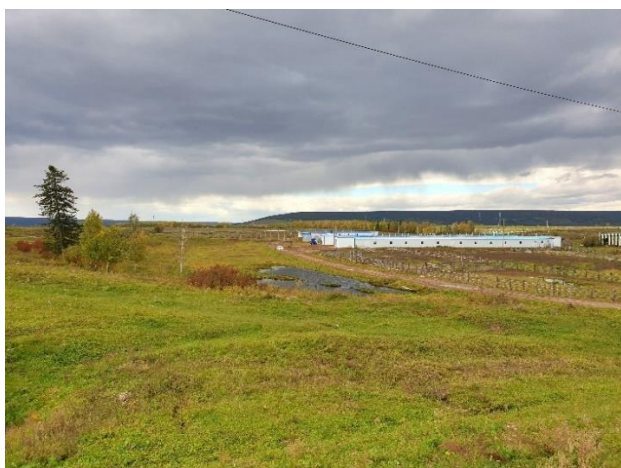
Fig. 42. Farm building of Kladovaya Olekmy LLC, built on an area of permafrost with low ice content, Yunkyr, September 2022. Photo by A.A. Suleymanov.
